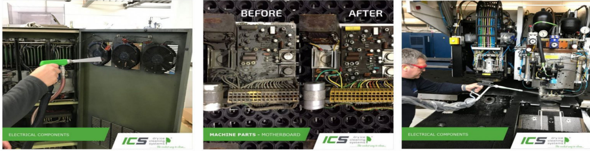
Figure 2 Use of Dry ice in Cleaning Purposes [6] "container-title": "ics-dryice.com", "title": "ICS", "URL": "https://www.ics-dryice.com/en/news/223/safe-way-of-electrical-equipment-maintenance", "author": [{"family": "Frio.sk", "given": ""}], "accessed": {"date-parts": [{"2025", 1, 20}]}, "schema": "https://github.com/citation-style-language/schema/raw/master/csl-citation.json"
